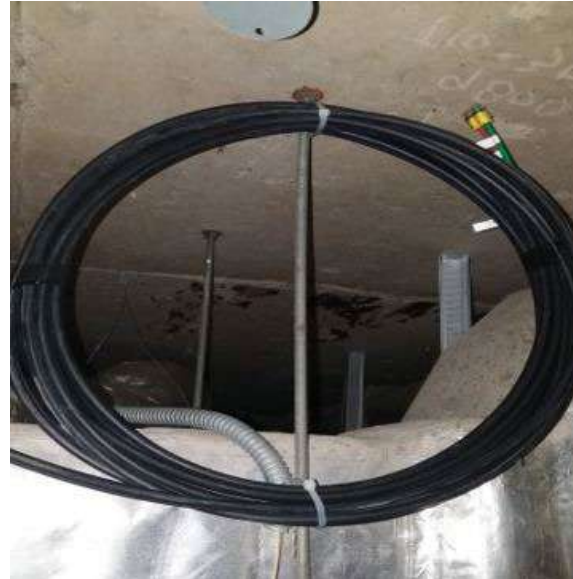
Photo shows ABF Microduct Coiled near Shop front
